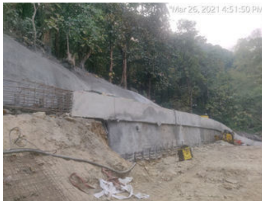
Photo- 4 (a) & 4 (b)- Casting of capping beam and micro-pile wall support with wiremesh and shotcrete and installation of deep drains and Installation of Permanent anchors after drilling
