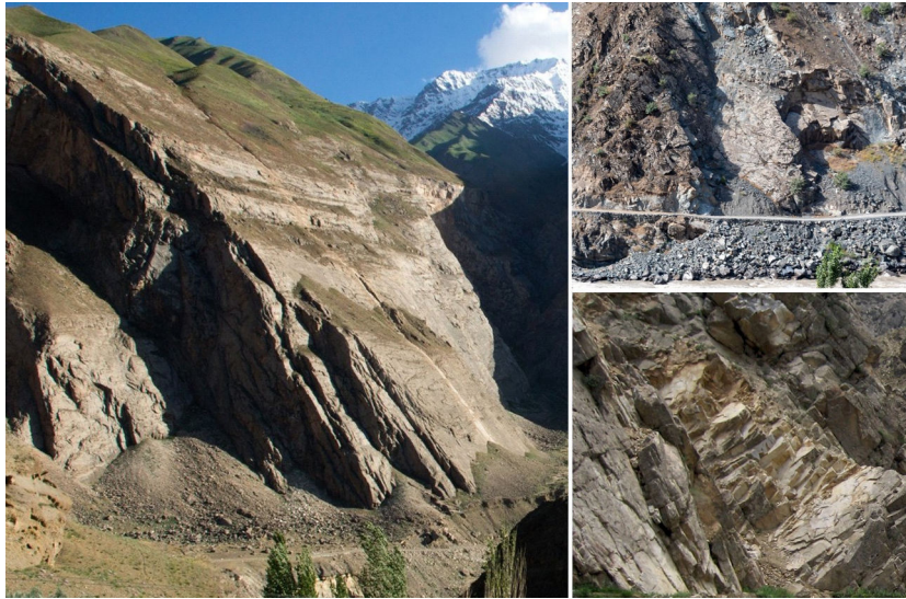
Figure 8. Slope failures belonging to Category III involving planar or wedge sliding
