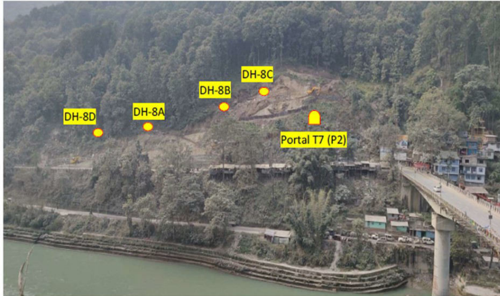
Photo- 2 (a) - Geotechnical Investigation: 04 nos. borehole along slide zone to establish the rock line for remedial measures
