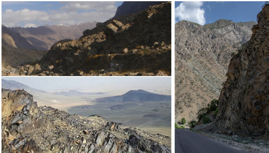
Figure 9. Slope failures belonging to Category III involving columnar toppling.
