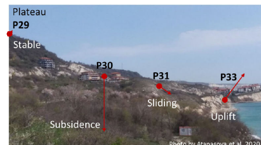
d. Landslide area shot from the west
