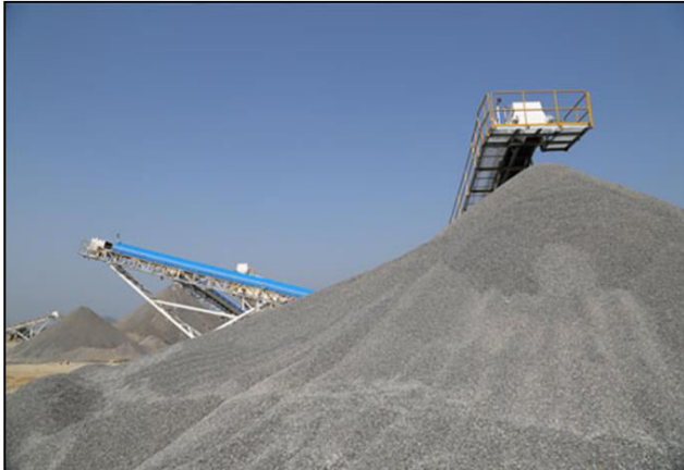
Figure 3. Local limestone aggregate trituration facility.
