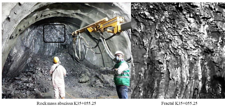
Figure 7. Fractal Dimension analysis of GGE Tunnel, Abscissa km 35+055.25
