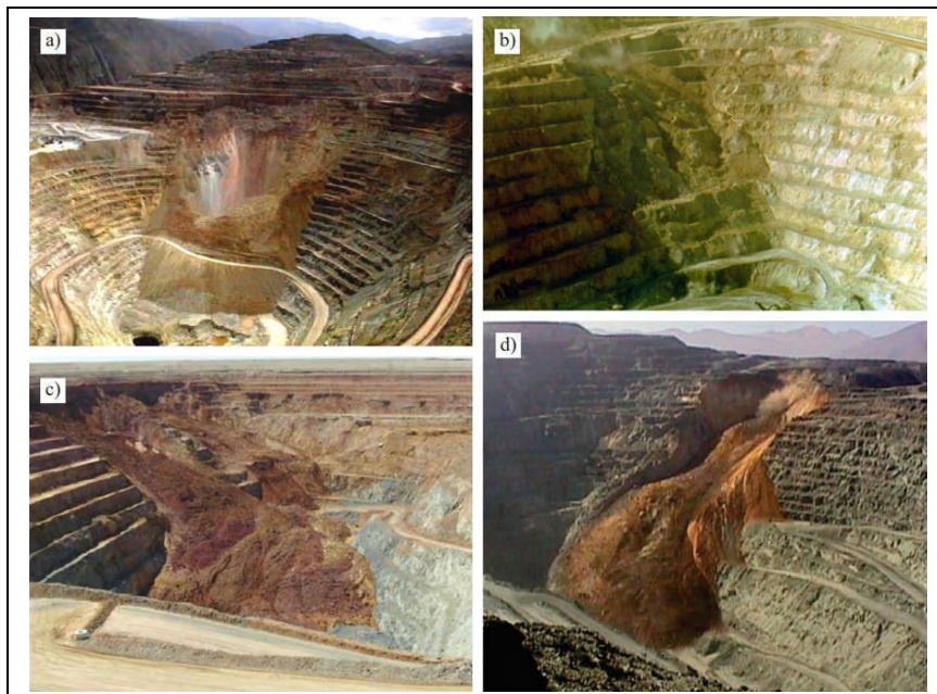
Figure 34. Four major open-pit failures reproduced by Carranza-Torres (2021).
