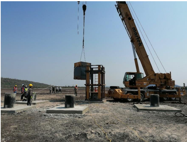
Figure 4. Image of the tests performed on site
