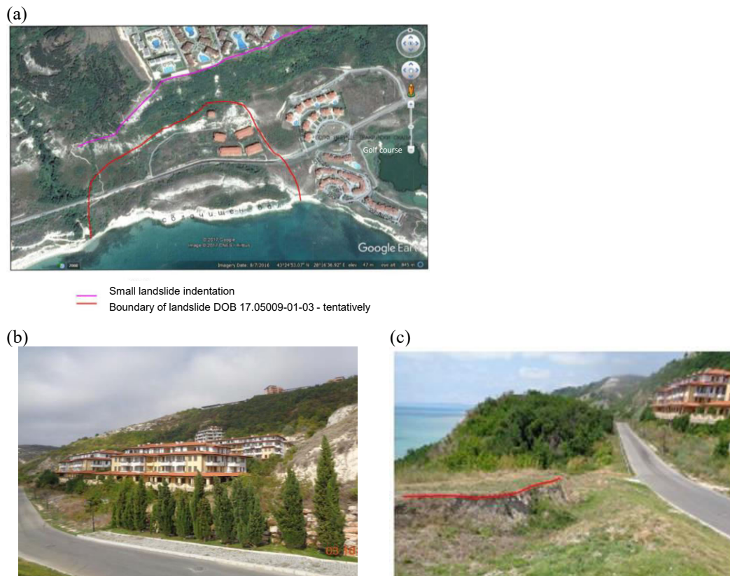
Figure 28. Landslide around eastern end of Topola village: (a) boundary of landslide body, (b) damaged buildings, and (c) transverse ridges (red line) (Министерство на регионалното развитие и благоустройството 2017, 2018, 2019).
