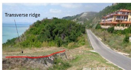
c. Transverse ridge of landslide boundary
