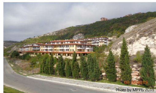
b. Buildings in landslide area
