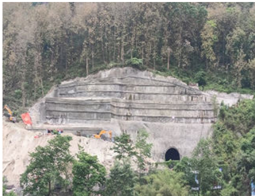
Photo- 5 (a) & 5 (b)- View of slide protection after several level of supports and View of active slide after slope support
