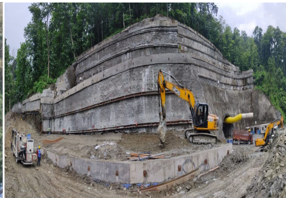
Photo- 5 (a) & 5 (b)- View of slide protection after several level of supports and View of active slide after slope support
