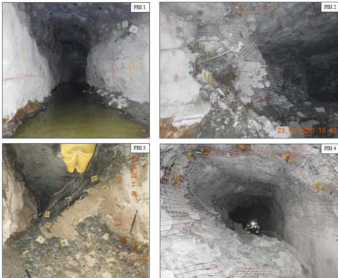
Figure 8. Examples of different Perimeter Burst Index damage classifications.
