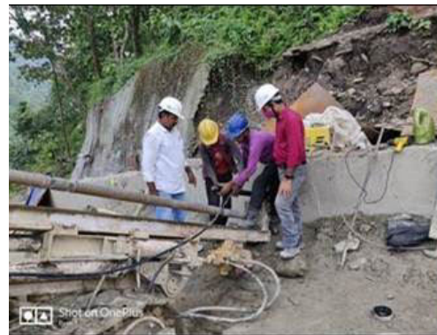
Photo- 4 (a) & 4 (b)- Casting of capping beam and micro-pile wall support with wiremesh and shotcrete and installation of deep drains and Installation of Permanent anchors after drilling
